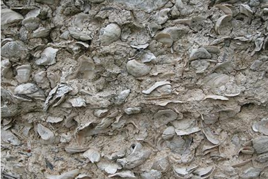
Close-up of wall
